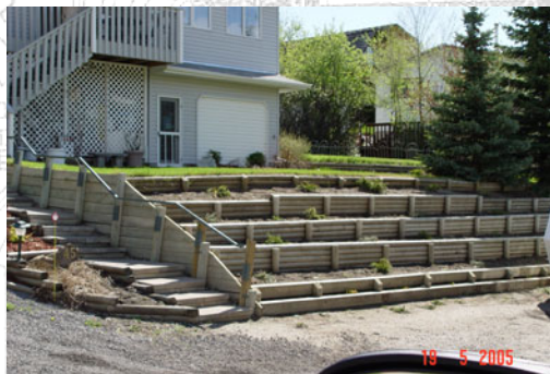
Figure 20: Hillside Retaining Wall System
