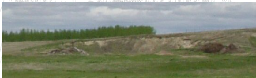
Figure 18: Sheet Erosion after Excavation
