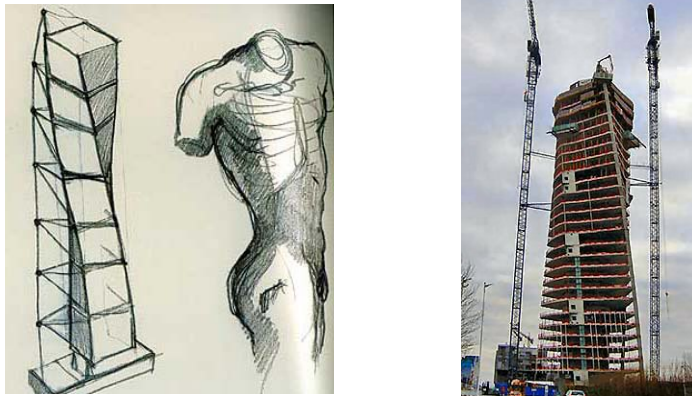
Figure 7: The Turning Torso, Santiago Calatrava, 2004
